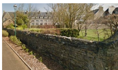
Muret - Roscoff - Source : Google Street View
